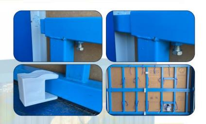
Tie (double knot) all the blue webbing around bulkhead frame.
