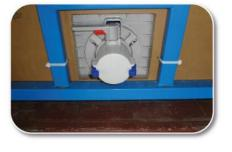
Valve needs to centered in the bulkhead aperture. Valve should arrive in the closed position.
